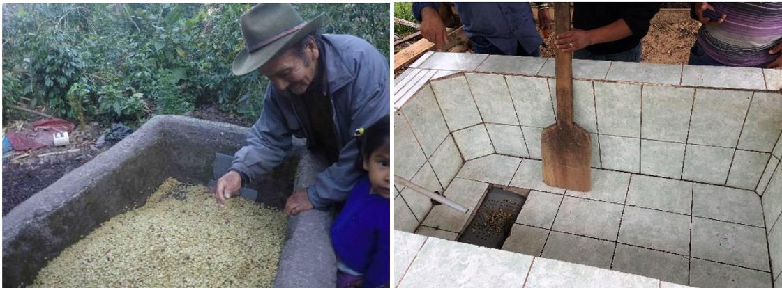
*A degrading cement fermentation tank on the Left and a new tile lined fermentation tank on the Right.*
